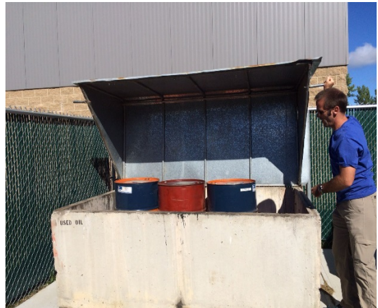
Proper outdoor storage of used oil containers – containers are protected from precipitation and are stored on an impervious surface.
